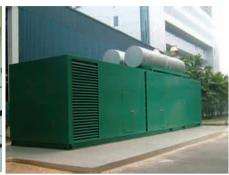
building monitoring system and providing new cabling system and fuel transfer system for 1 set of 2MVA and two existing 1.25MVA generator sets.
